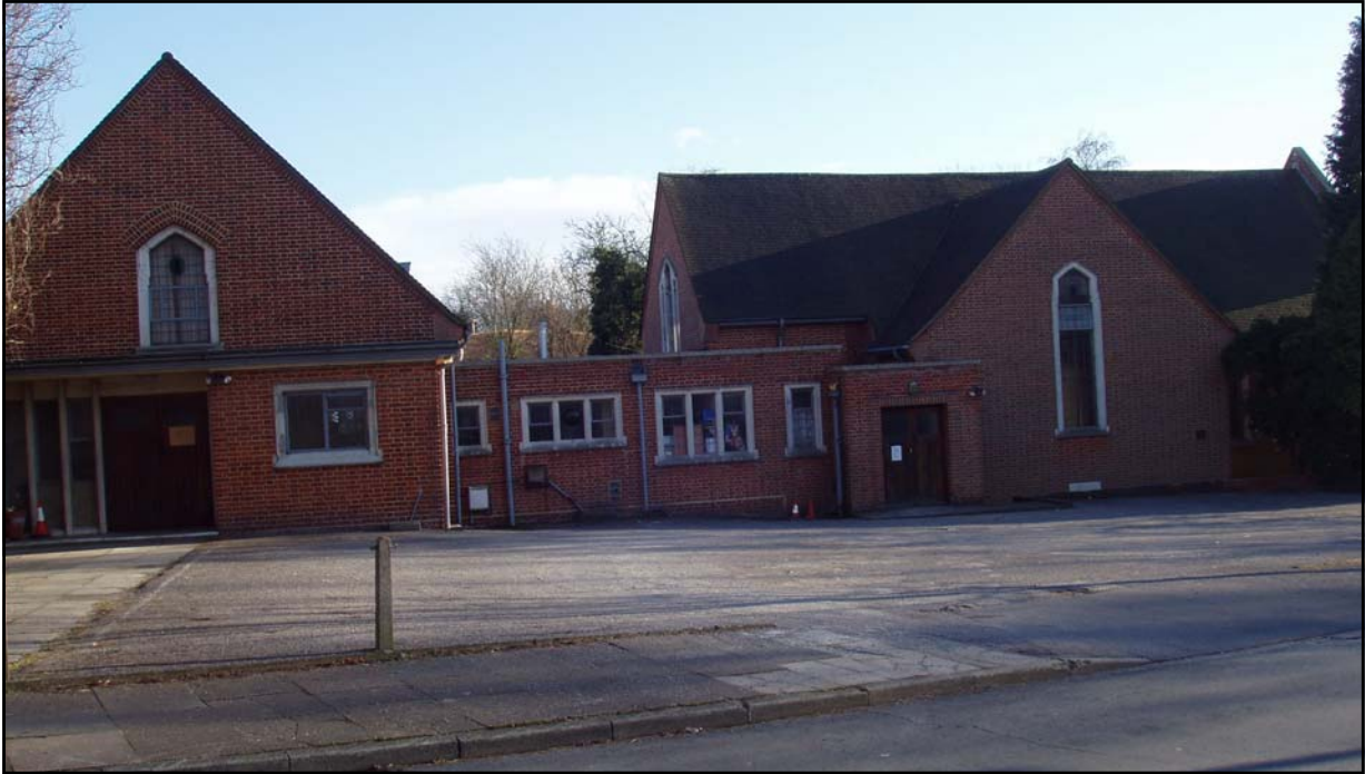
Inappropriate treatment to the car park of Eastcote Methodist Church
