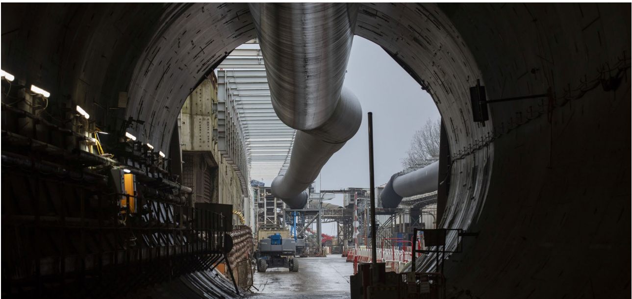
The conveyor structure leaving the West Ruislip Portal on its way to the treatment area at Harvil Road
