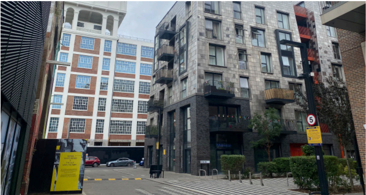
View between new residential building and Power House towards the Cabinet Building
