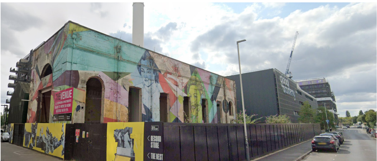
Hoarding around the Power House
