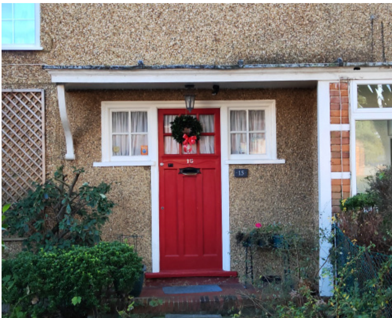
15 Morford Way, original door and porch
