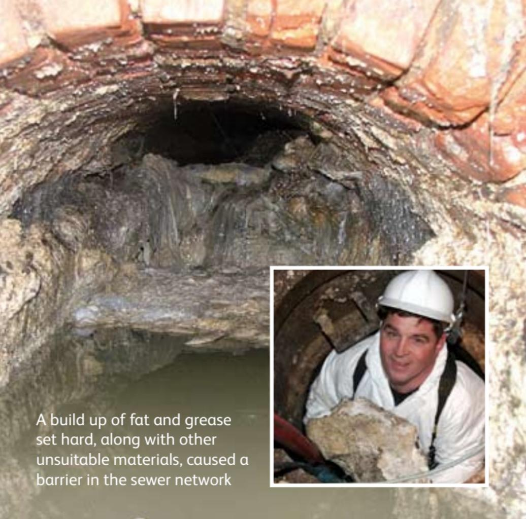
A build up of fat and grease set hard, along with other unsuitable materials, caused a barrier in the sewer network
